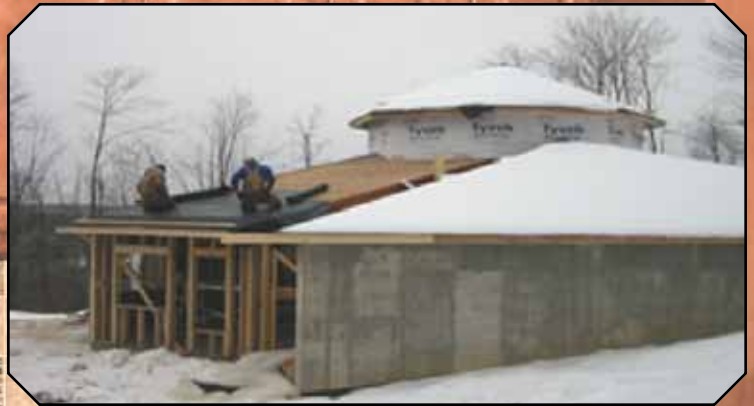
On-Site Built Building Weather
